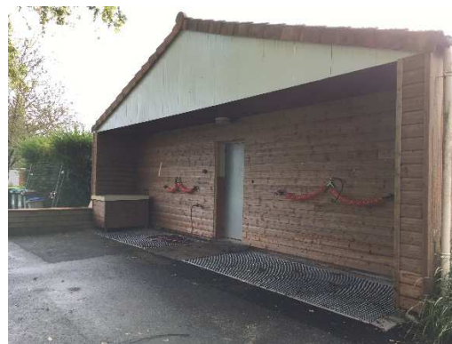
Travaux station lavage
